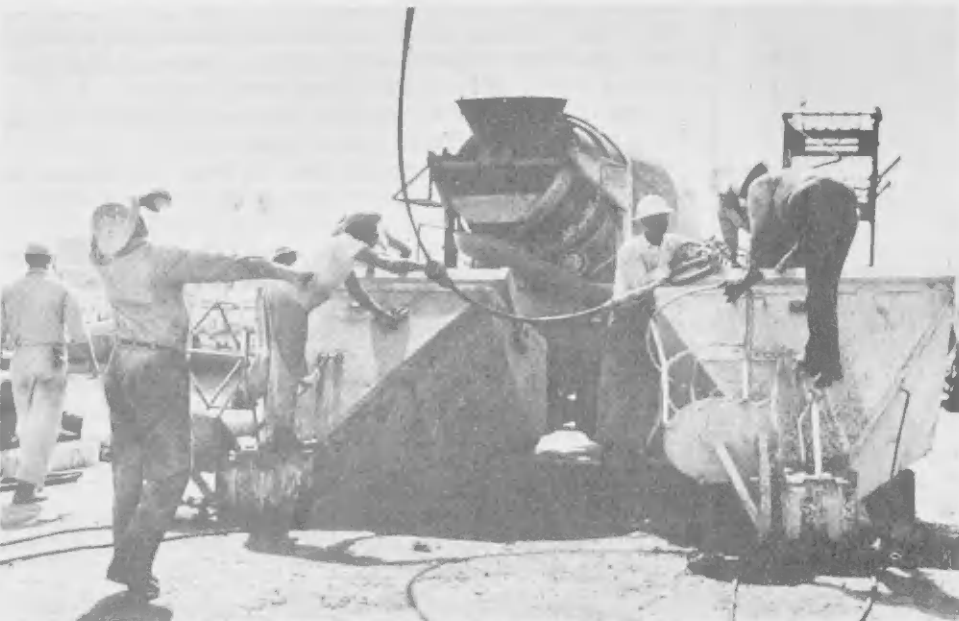
THREE READI-Mix trucks kept concrete hoppers, above, continually filled in the dawn to dusk operation. After a two-cubic-yard hopper, left, was filled, it was swung out to the dolphin by Raymond's big crane, lower left, and dumped in the steel reinforced base, lower right.
